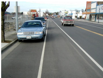
The photo above shows how a stripe can be placed to create a “buffer” or safety zone between the parked car and the travel lane. The photo below shows the principle of a colorizing the buffer area for greater distinction between the buffer and travel lane.
