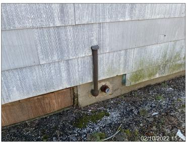
**Photograph 3.** Fill and vent piping protruding from the foundation wall in the northwestern portion of the building, adjacent to the driveway.
