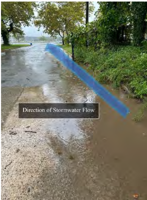
Exhibit C. The former roadway existing within the southeast portion of the site directs stormwater into a Municipal Separate Storm Sewer.
