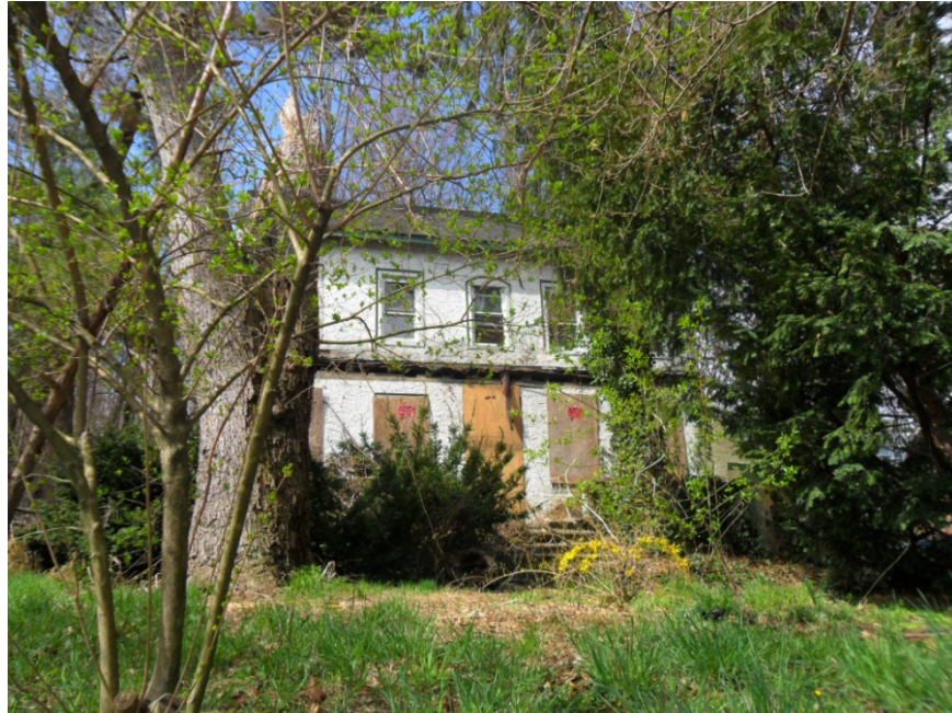
Photograph 17: Abandoned building; view looking west from near Community Drive
