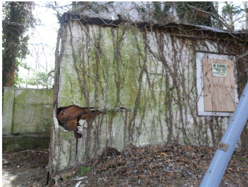
Photograph 22: Abandoned building; view looking south
