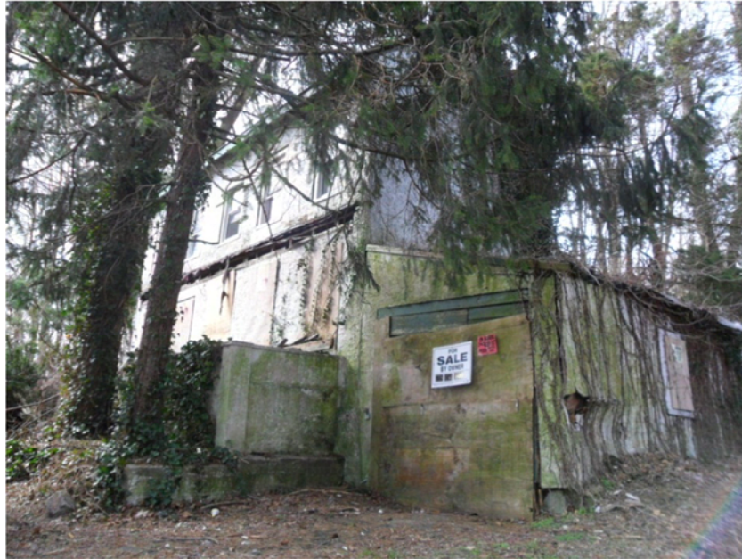
Photograph 21: Abandoned building; view looking west
