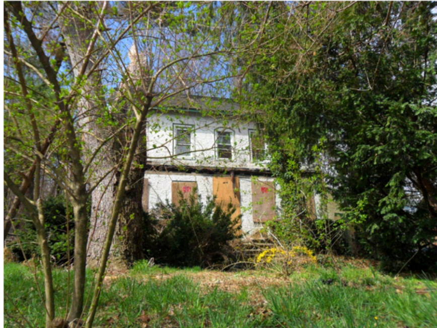
Photograph 25: Abandoned building; view looking west
