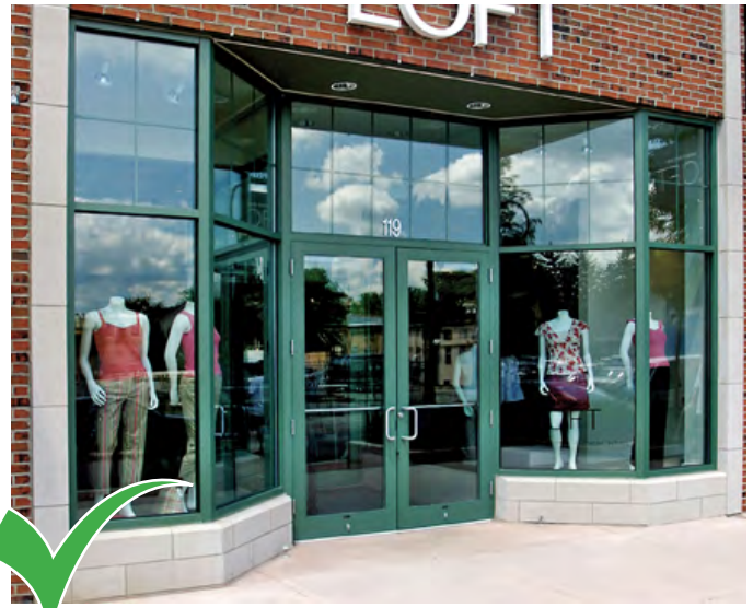
Do use aluminum windows with a finish matching the color scheme of the building.
