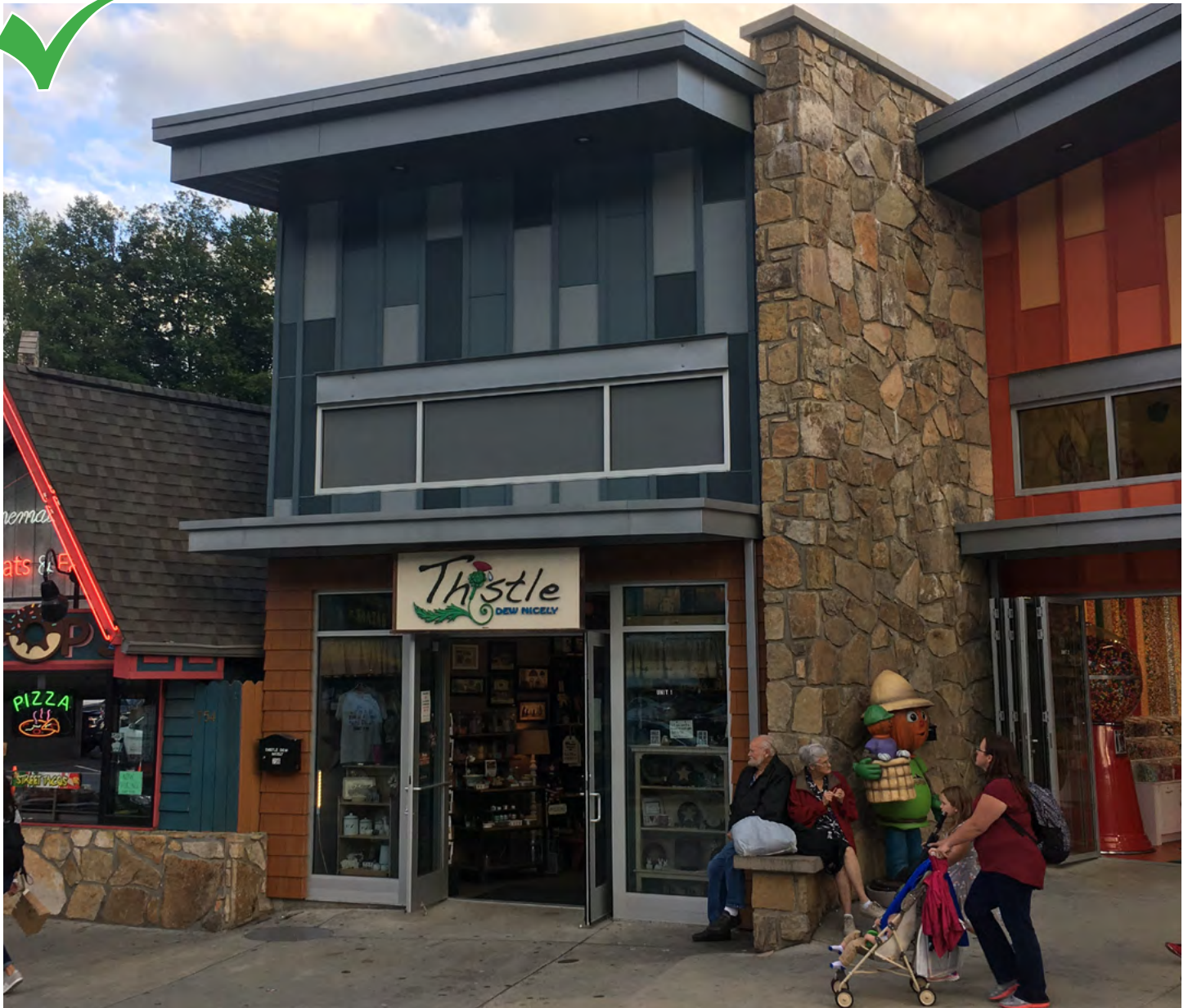
Use materials that can be repaired and maintained - such as fiber cement panels and siding.
