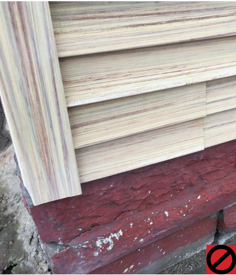
Do not use residential vinyl siding or paint a fake wood grain on it to mimic wood siding.
