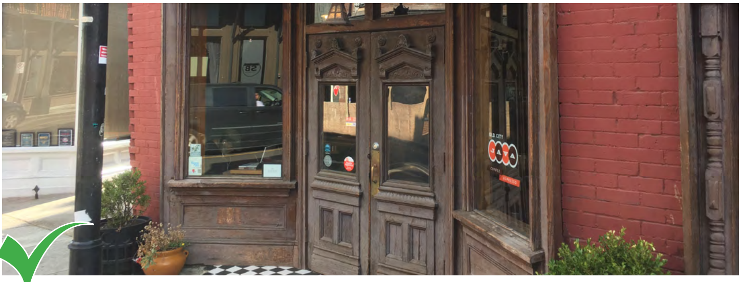
Use and maintain wood details when appropriate, such as storefront windows and doors.
