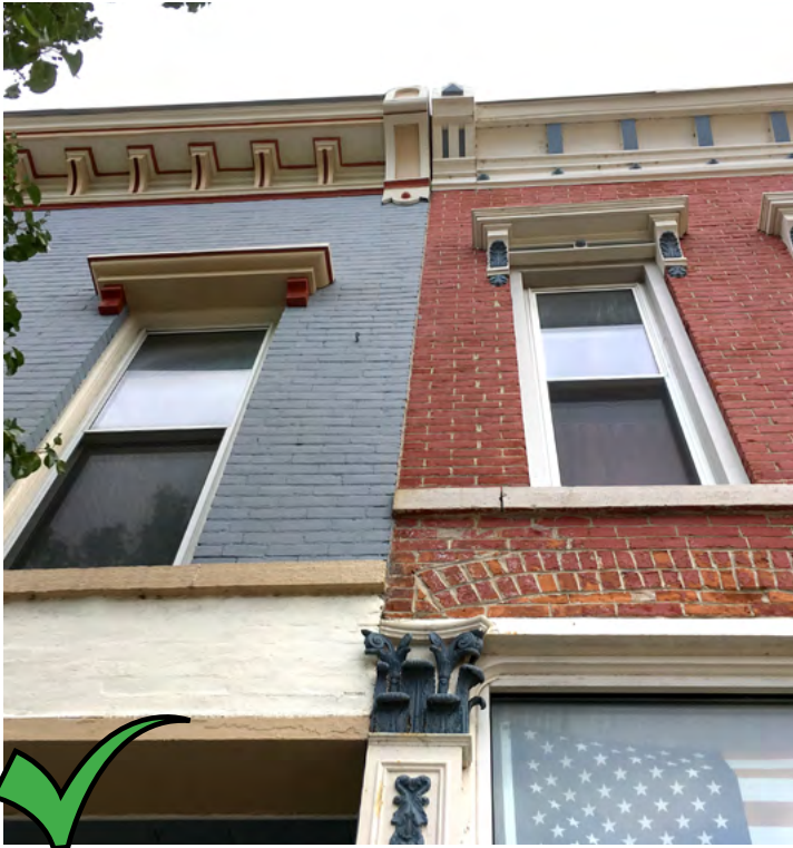
Do restore and highlight cornice lines, corbels, door & window lintels.
