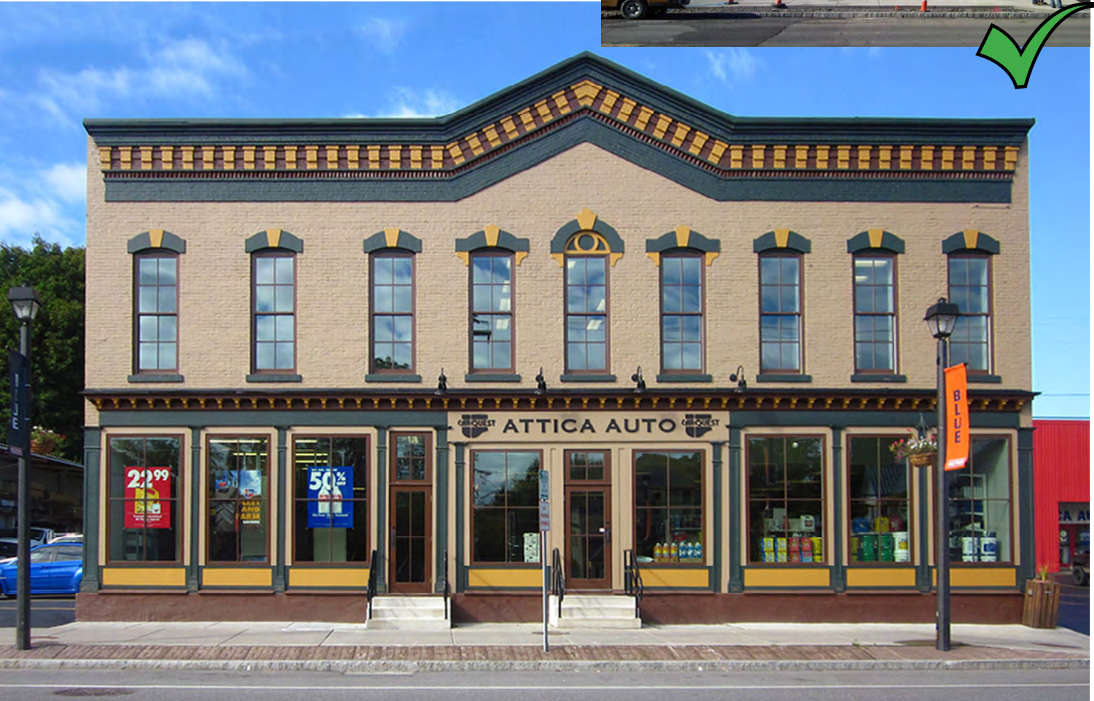
Do restore original window openings that have been covered over - and detail masonry with color.
