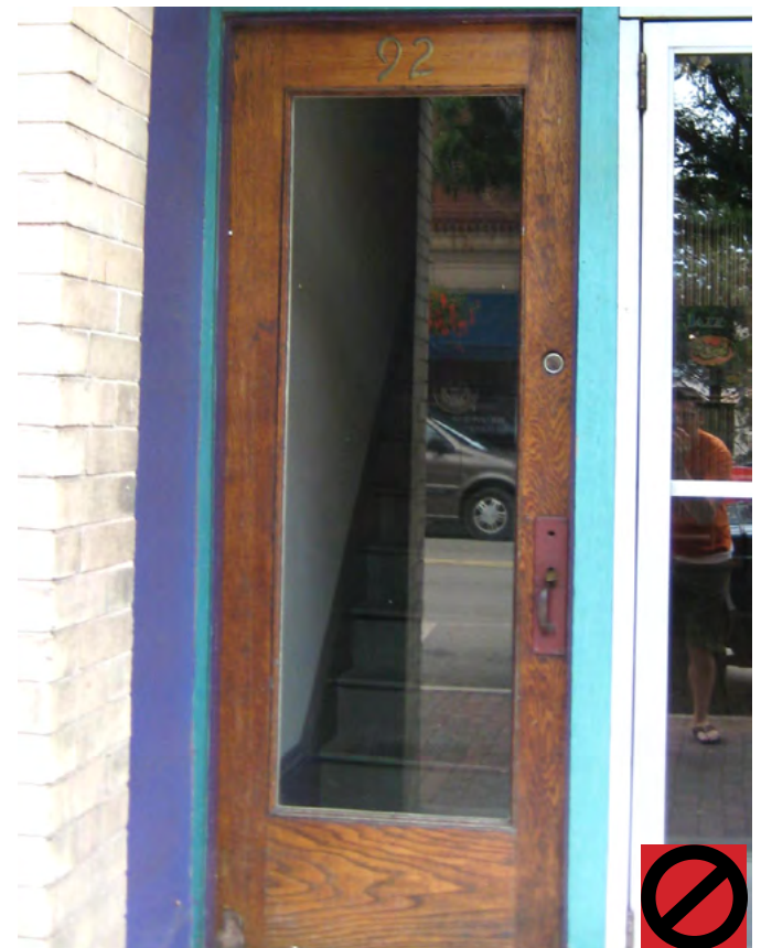
Don't use full glass entry doors for upper floor residential - It can appear as a commercial entry.
