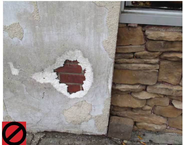
Do not use EIFS to cover original materials or in places requiring increased durability.
