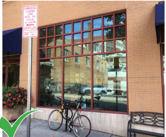
Do use a variety of window patterns and sizes to bring down the scale of large openings.
