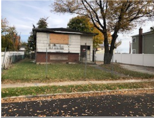
Figure 3 212 Sheridan after clean and board
